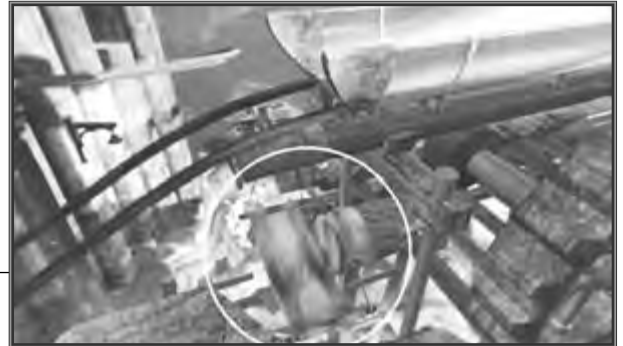
Fig. 4-8. Note the sling-like basket (circled here) hanging from this near end of the bridge.
