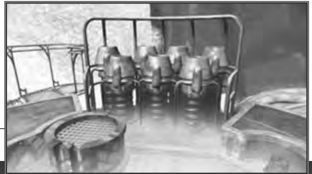
Fig. 6-6. These circuit coils mean electricity is nearby. In fact, a generator powered by geothermal vents is below you.
