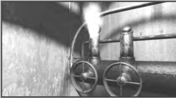
Fig. 3-40. When a valve cap is up and venting air (as seen here), the valve is "open."
